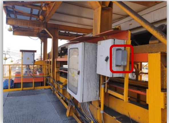
All these parameters were incorporated in the development of the RFID input card reader using low-power operation and the SIGFOX IoT network adapted to it. Thus, the worker has a reader available in the vicinity of the controlled technology to which he attaches his input card. By pressing a button on the device, he then simply activates its reading and sending it over the wireless network to the tracking center. Once the
