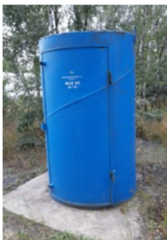
Figure 2 Steel container above the borehole
