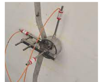
Figure 6 Crack measurement in construction with 3 probes
