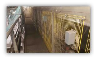
The plant operation receives information via SMS when a temperature spike is detected (warning message) or a critical temperature value is exceeded (alarm message). Upon receipt of the alert, the maintenance staff checks the condition of the rollers in that
